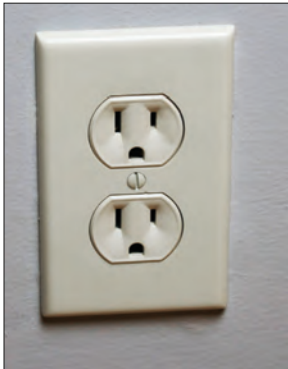
Figure 1.4. A standard receptacle in American homes is rated for a current of 15 amperes.
